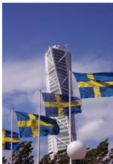
The Turning Torso Tower in Malmö
